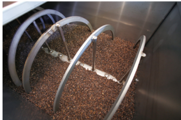
Inside the waste treatment tank human waste is mixed with buckwheat chaff.
